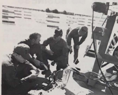
Sgt. Robert Benton, TSgt. Charles Phillips, SSgt. Dewey Beene and Sgt. Jack Hesselstine perform a guidance system check on a AGM-65 Missile before releasing it to be uploaded on aircraft.
